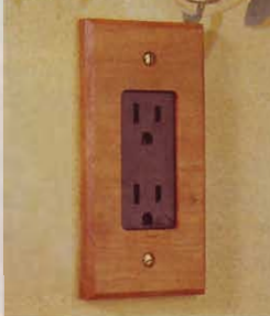
A We oriented the grain horizontally on this cherry wall plate.
